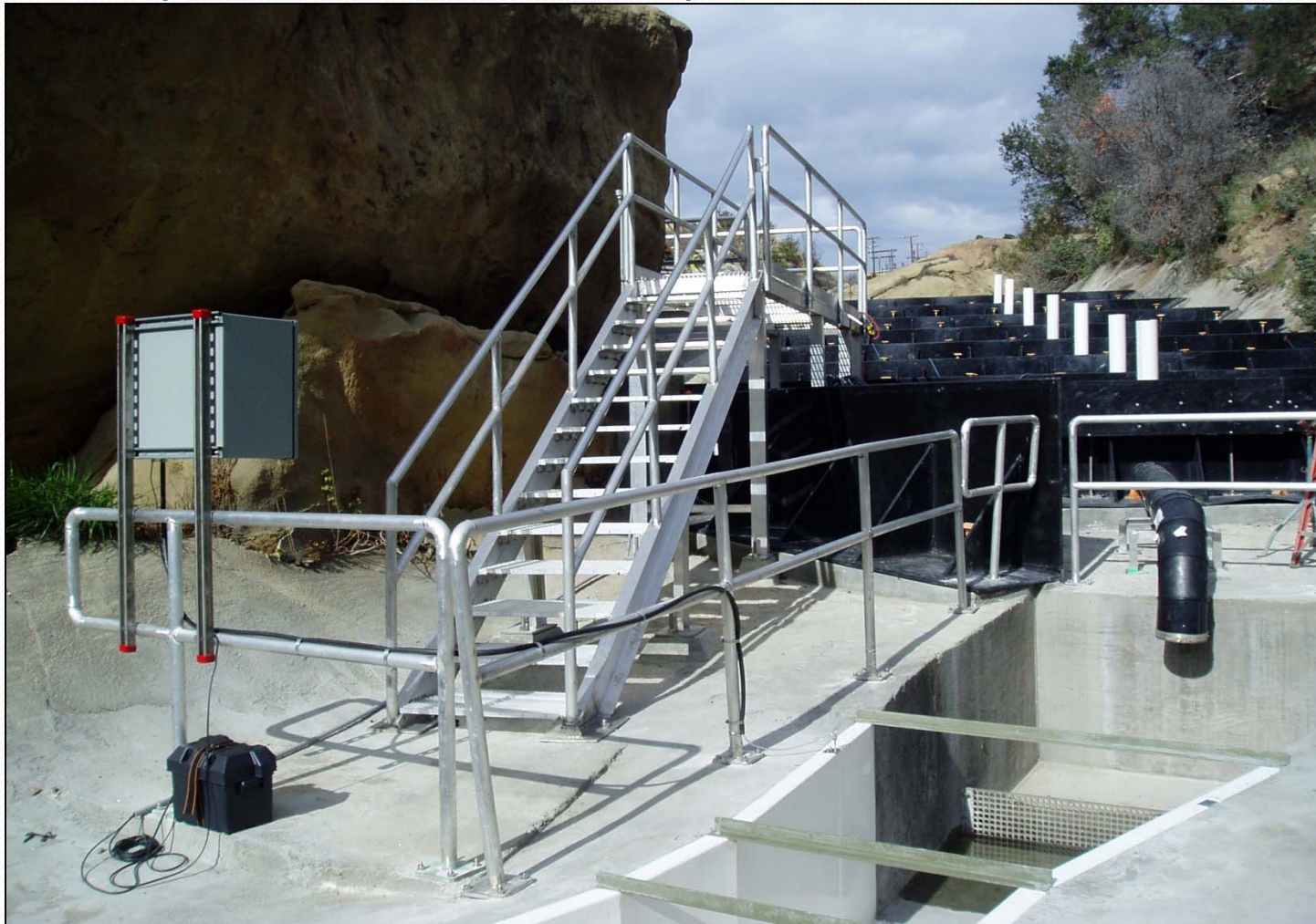
Upstream View After Multiple Filter Bed Installation
