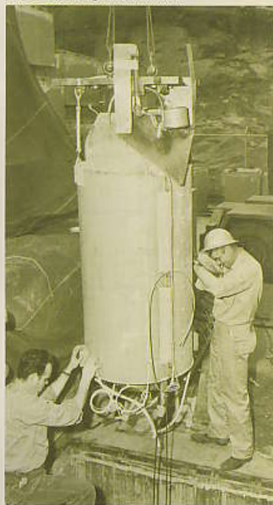
43 Hot Trap Installation.
