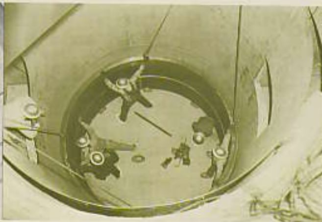
12 Thermal Shield Rings of cast steel, 5-1/2 inches thick, are being lowered into place inside the outer tank. The rings are not welded to each other and the bottom ring simply rests on the bottom of the outer tank to permit free thermal expansion.
