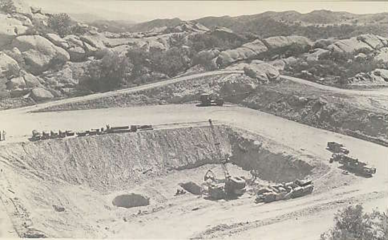
2 Site Excavation, March 1955. The circular cavity to the left will contain the foundation for the reactor core; those to the right are for the fuel storage cells, the fuel element cleaning cells, and the hot cell.
