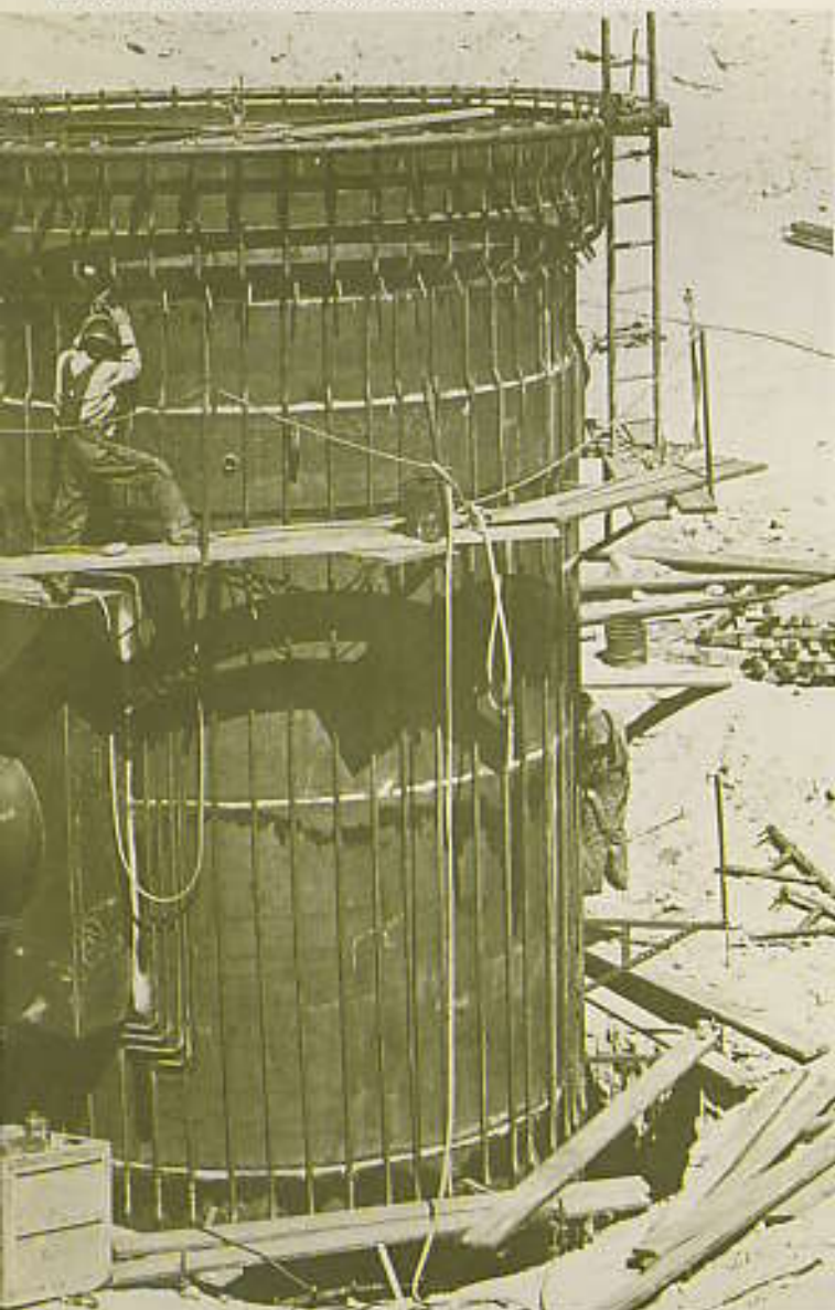
9 Cavity Liner of the reactor core, showing the tetralin coolant lines to remove heat from the concrete shielding which will surround this tank. The large hole, left of center, will contain the sodium inlet and outlet pipes.
