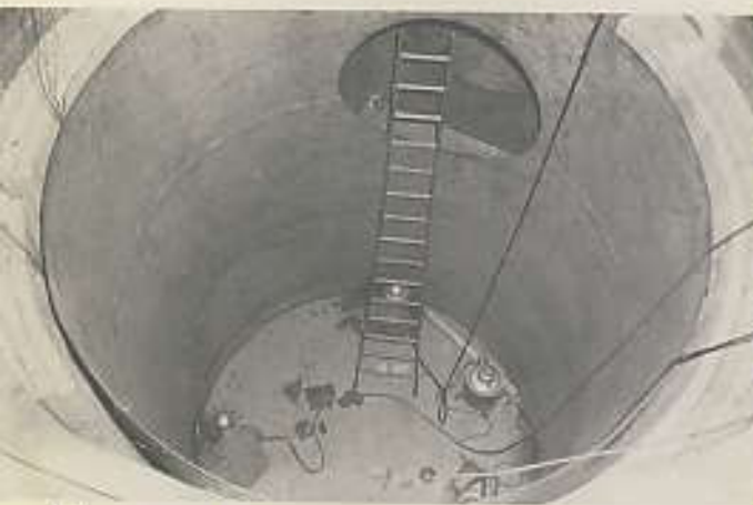
11 Outer Tank of 1 4-inch-thick, low carbon steel will contain the sodium in case of a leak in the core tank. It is 12-1 2 feet in diameter and 19 feet high.
