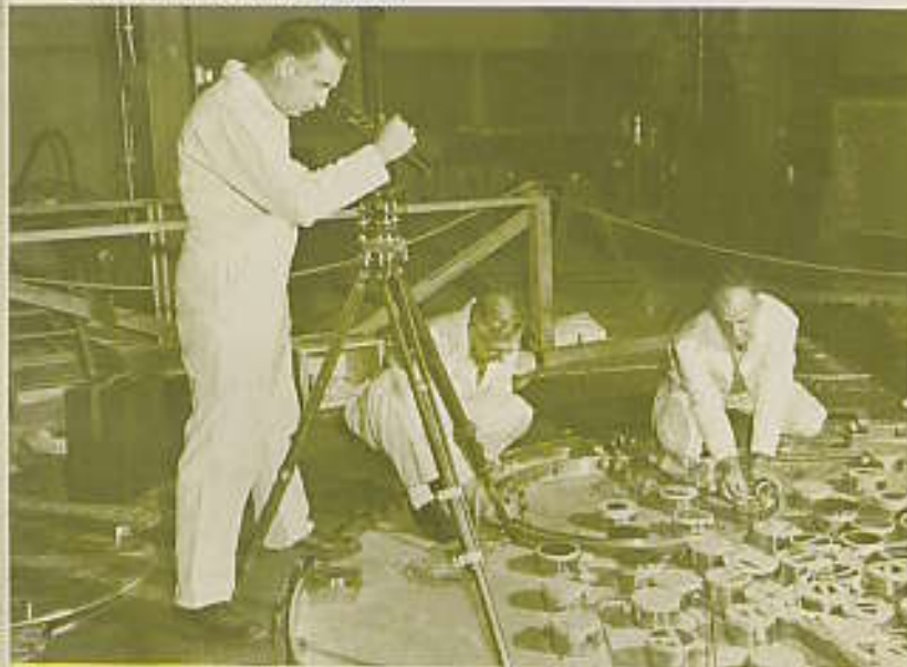
22 Checking Alignment Of The Reactor Loading-Face After Installation.
