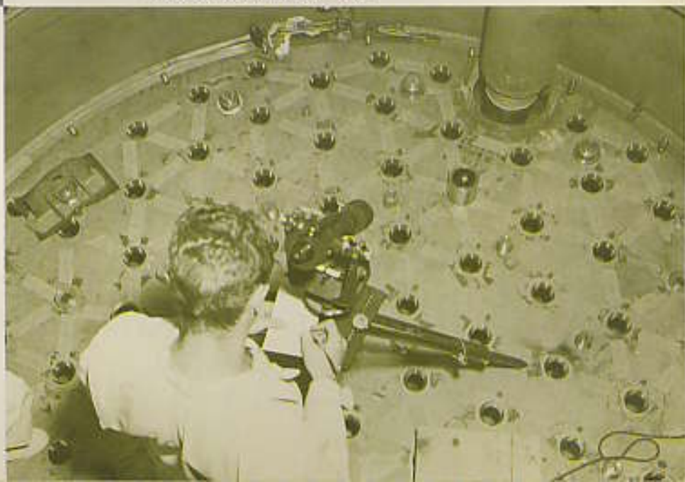
15 Bottom Grid Plate inside the core tank. Sodium enters the core tank into the plenum beneath this grid plate. Pedestals at the bottom of each canned graphite moderator assembly fit into the holes in this grid plate, thus positioning the can. In addition, the pedestal has a circular channel along its axis which directs the sodium from the lower plenum up through the coolant tube in the moderator can assembly.
