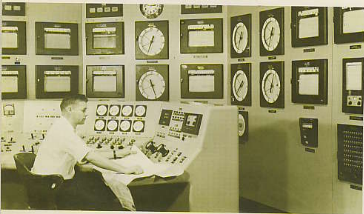
27 Control Room. showing control console and a part of the bank of recording and indicator instruments.
