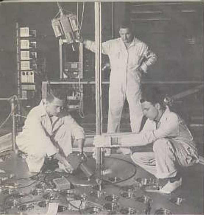
23 Experimental Loading Of SRE Fuel Element into core. The element is made up of seven rods, each rod consisting of twelve 8-inch long uranium slugs, in a thin-walled stainless-steel jacket-tube. The six outside rods are spirally wrapped with stainless-steel wire to maintain spacing between the rods and to assure mixing of the sodium as it flows through the inner passages just surrounding the central rod, and through the outer passages surrounding the six rods. At the bottom of the rods is a locating guide and an orifice plate for controlling the flow of the sodium as required for each particular coolant tube. The entire fuel element is attached to a plug in the loading-face shield by a hanger rod.
