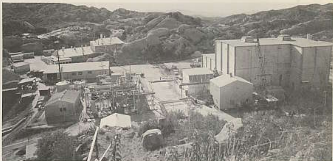
6 SRE Site at completion of construction in March, 1957, at which time pre-operational tests were already being carried out. The large building to the right of the photograph contains the reactor and its associated equipment and controls. The structure immediately to its left is the sodium-air heat exchanger. From the reactor building, sodium piping leads across the roadway, left, to the steam generator of the electrical generating plant. At lower left is the power plant control building. Other buildings shown in the left center part of the photograph are engineering development laboratories.
