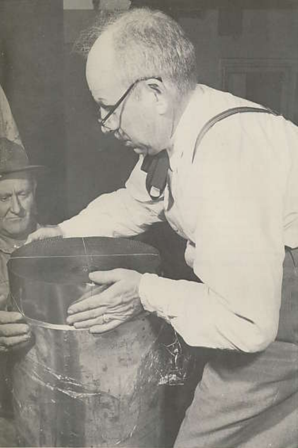
42 Corrugated Zirconium Foil being inserted into the hot trap during construction.
