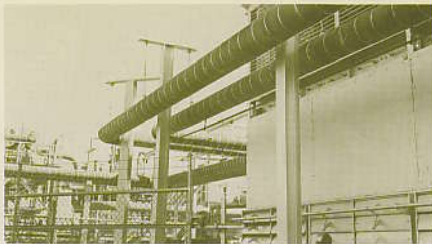
44 Secondary Sodium Lines lead out to the steam-electric plant. These lines are 8 inches in diameter and carry nonradioactive sodium to the steam generator at 900° F and 50 pounds per square inch absolute, returning the sodium at 440° F. The sodium velocity is 13 feet per second.
