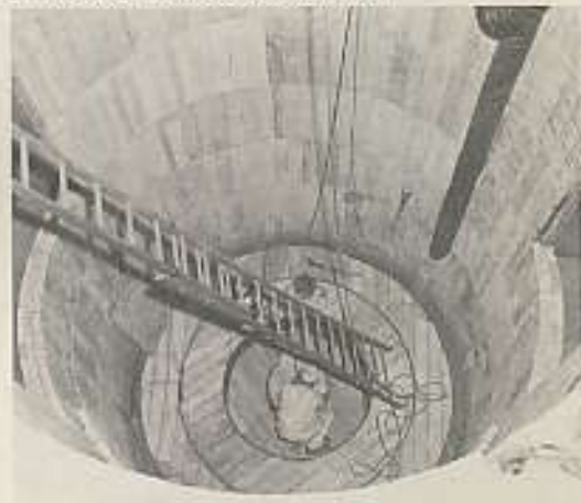
10 Thermal Insulating Blocks being installed inside cavity liner.
