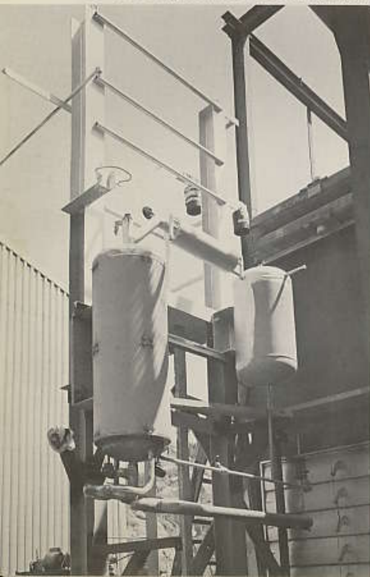
40 Cold Trap installed in secondary system.
